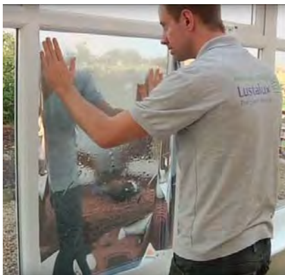
Reflective or Low-e window films: Manufacturers provide step-by-step instructions for installing their products.
