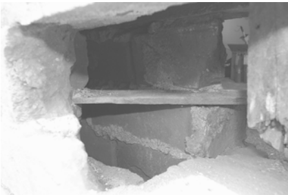
Hollow brick wall: Two separate single brick walls are held together by wood lath embedded in the mortar joint.
